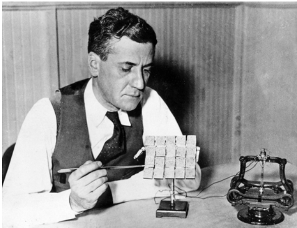
FIGURE 5. Rhamstine demonstrating how selenium cells could power a motor in 1935.
